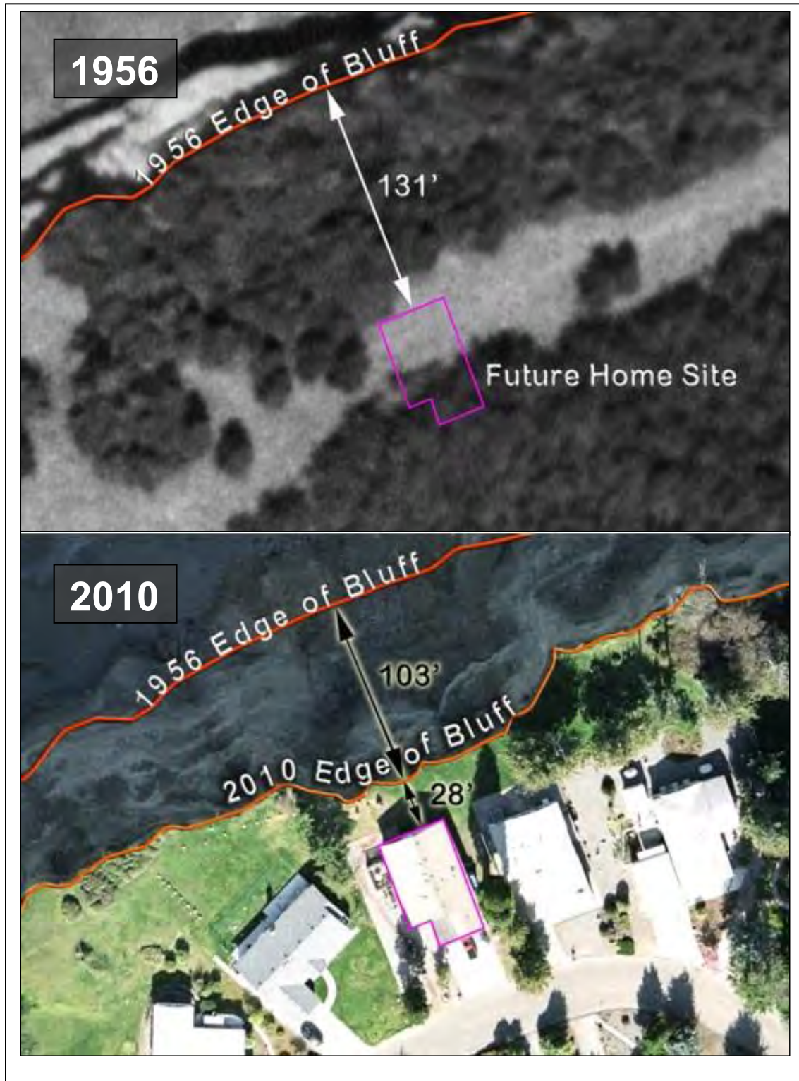
Figure 1-8. Bluff erosion threatening homes along Cypress Circle, west of Dungeness Spit (Source: R. Johnson)
