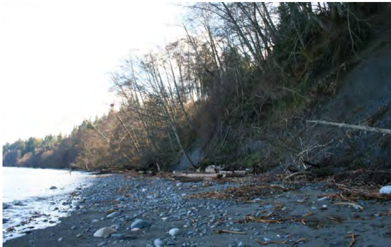
Figure 1-9. Erosion at base of bluff contributing sand, cobble and gravel to the nearshore. Erosive forces could become more severe in the future due to climate change (Photo by A. MacLennan)
