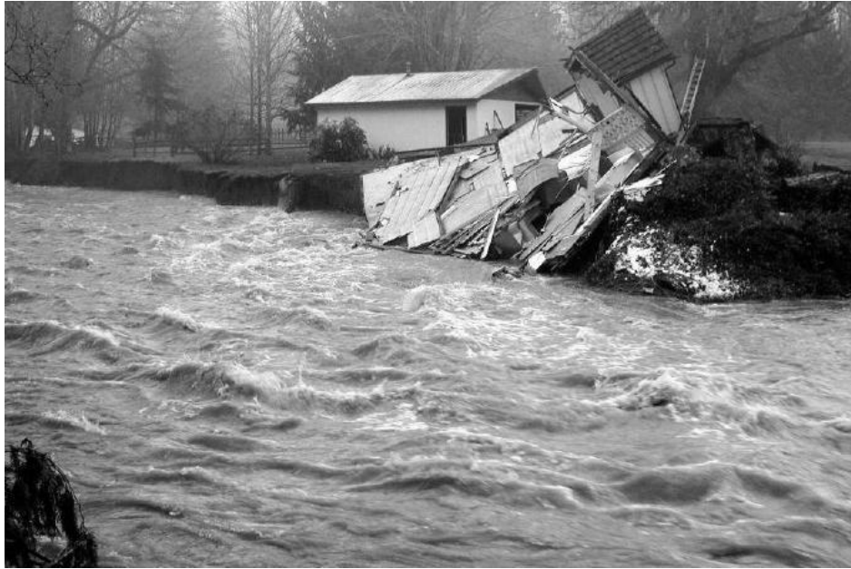
Figure 1-12. Locating new developments outside of channel migration zones will help prevent situations like this which occurred during a recent Dungeness River channel migration event (Photo: Randy Johnson)
