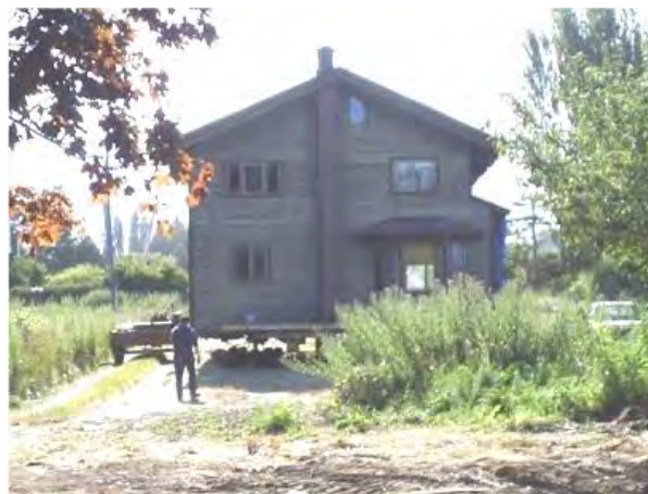
Figure 1-13. The County and partners are moving existing developments outside of channel migration zones to prevent potential human and property harm; this project along the Lower Dungeness River also allowed for riparian and floodplain restoration (Photo: Clallam County)
